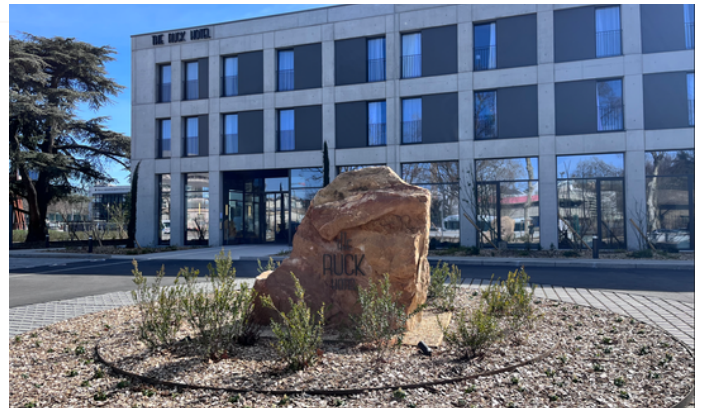
THE RUCK HOTEL 345 AVENUE JEAN JAURÈS 69007 LYON TEL : +33 (0)4.28.38.69.00 SITE : HTTPS://THERUCKHOTEL.COM/
